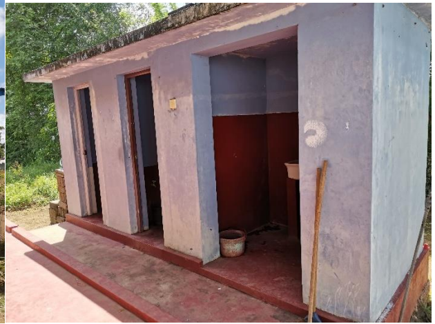
Existing toilet facility in the ASC
